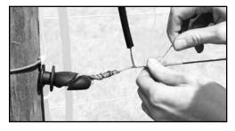
4. Connect the end of the insulated wire (from step 3) to the portion of the fence that is to be energized. Conductor line to be protected.
