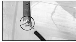
5. Attach an insulated wire to the bottom of the diverter.
