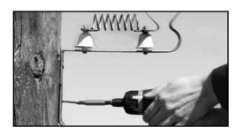
1. Using the two holes in the steel diverter plate—screw, nail or wire the diverter to a wood or steel post.
